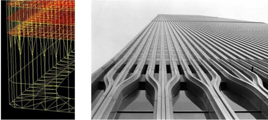
**Figure 1.1** Structure of ground floor facade for the FEA and corresponding geometry. The FEA abstraction cannot properly represent the complexity of the shapes, especially at their meeting points.
