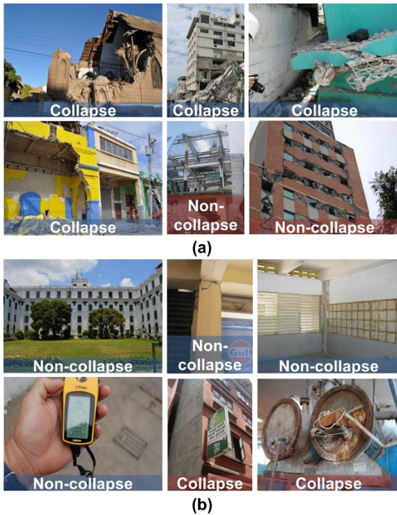
Figure 3. Examples of the collapse classification result: (a) classification of positive images and (b) classification of negative images. Note that the text labels indicate classification results, and blue and red colors are true and false classification, respectively (e.g. an image in (a) having a label of “collapse” in blue is true classification collapse building image)
